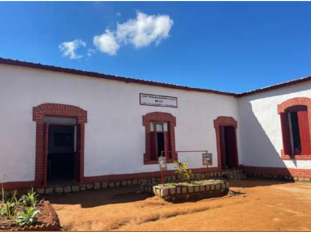
Building rehabilitation work
